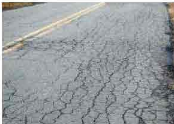
Figure 11-3 faïençage serré
