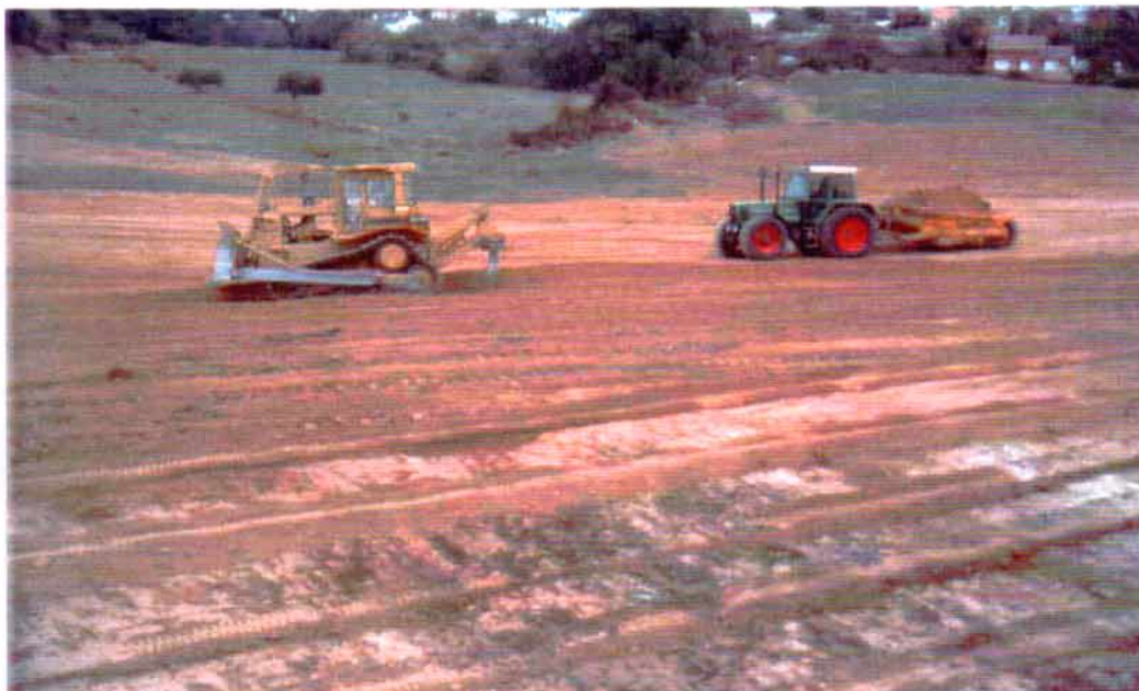
Figure 2.- Land surface mechanical reshaping for new vineyard planting pattern in Alt Penedés (Catalunya, Spain)
