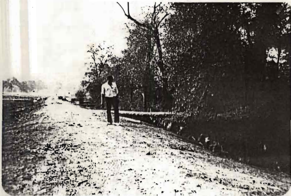
figure C.12: Barrage de Boudouck
