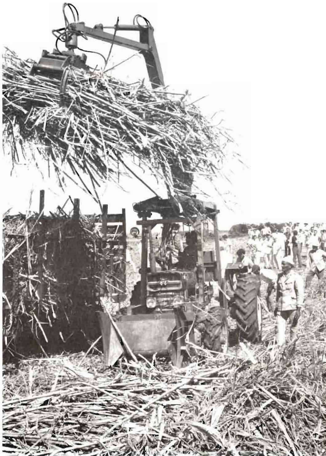
Plate V. Demonstration of SIMSON loader.
