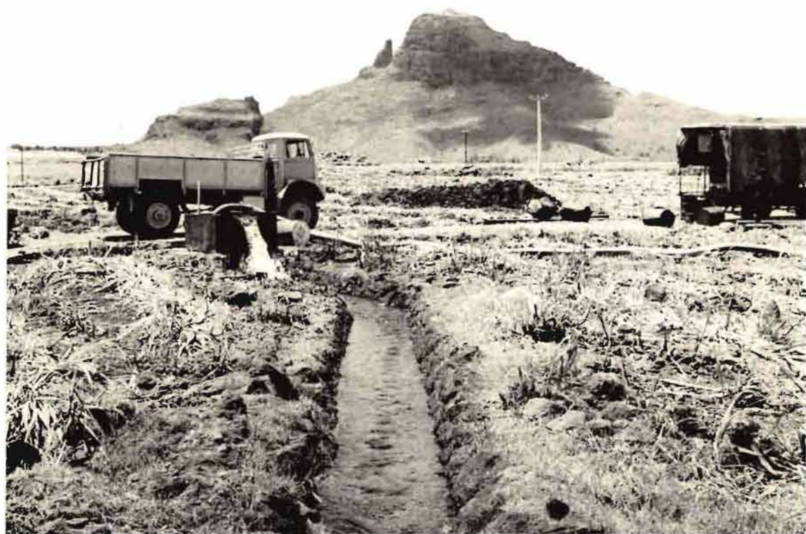
Fig. 13. Ground water research. Pumping tests in progress at Belle Rose ( above ) and Palmyre ( below ).
