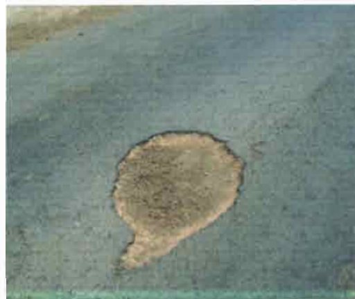
Figure III.20 : Nid de poule sur Notto-bayakh
